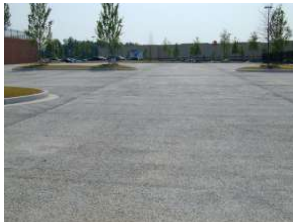
Pervious concrete can offer a durable, yet permeable, surface capable of supporting heavy traffic loads or design storm.
